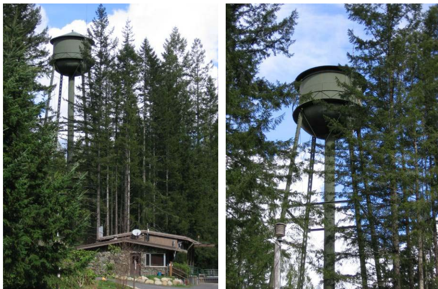
Elevated Water Tank (left photo shows the Treatment Building in the foreground)
