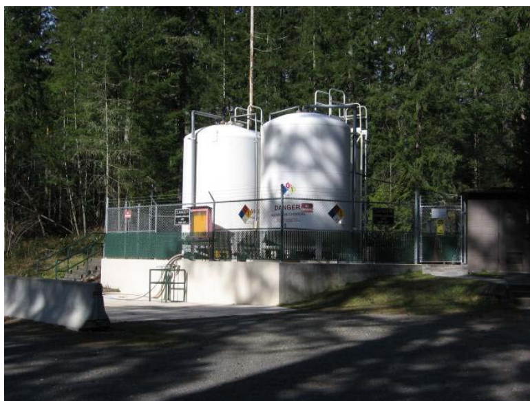
Fluoride (Hydrofluosilicic Acid) Storage at Landsburg
