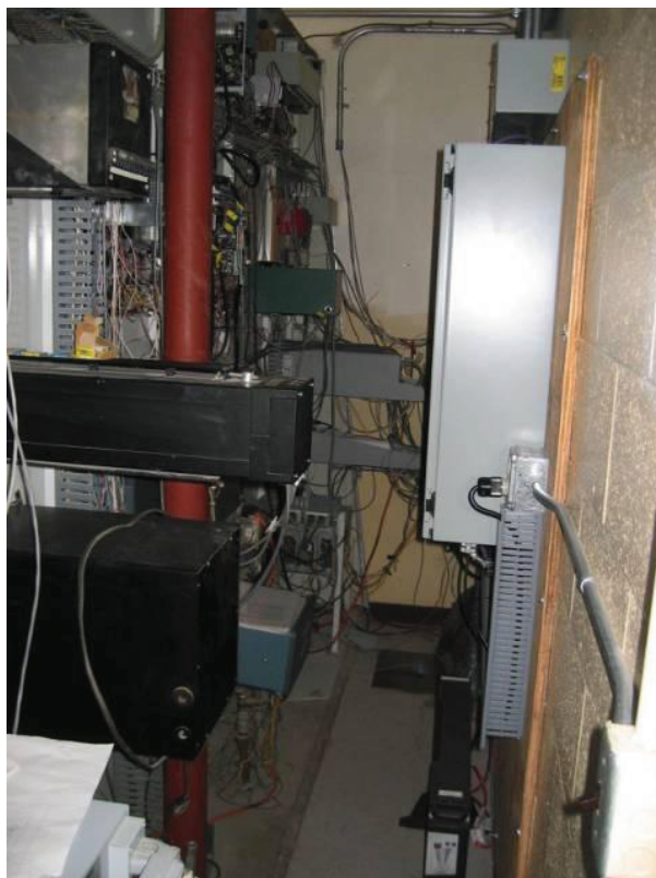
Photo 2-28. Treatment Building SCADA/Telemetry Space
