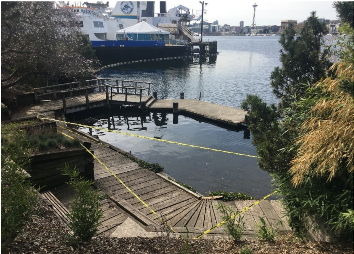
Park boardwalk, pier and float. Looking southwest.
